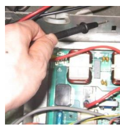
Figure 4-4.5: Measuring resistances between compressor terminals and ground
